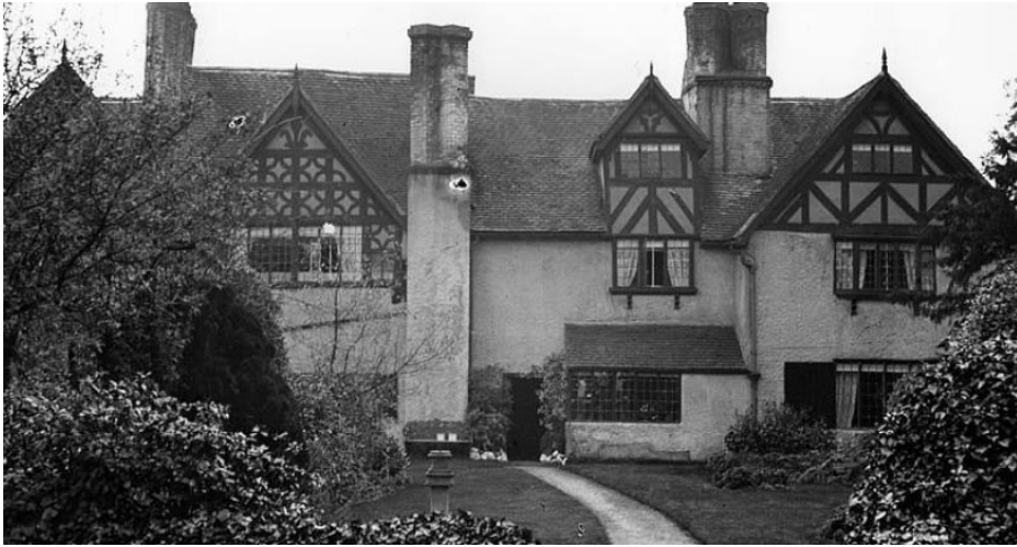
ii Handsacre Hall before demolition
